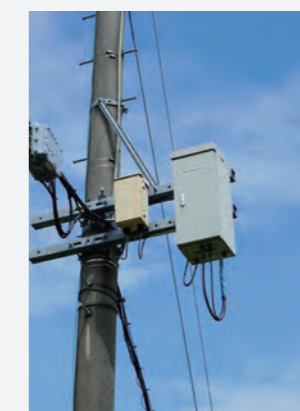
屋外用無停電電源装置(CATV/基地局用) Uninterruptible Power Supply Unit (for Cable TV transmission equipment)
